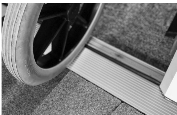
Low threshold demonstrated using a wheelchair
