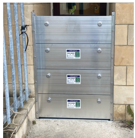
Photo shows Stop Log Barrier protecting a single main access door
