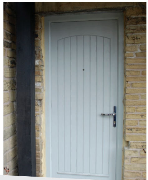
New flood screen & access door onto the Calder Hebble Navigation.
