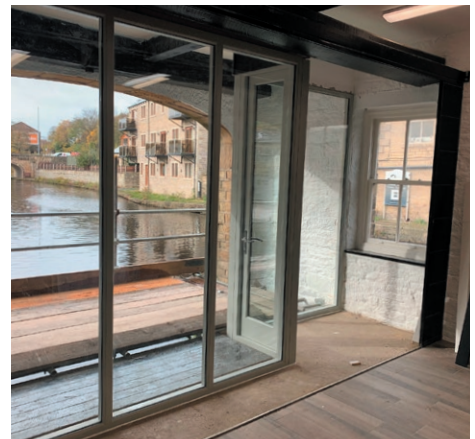
New flood screen & access door onto the Calder Hebble Navigation.
